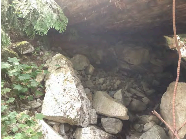
Right Bank Abutment when facing downstream
