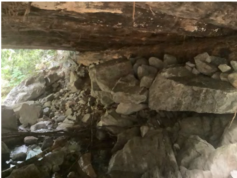
Right Bank Abutment when facing downstream
