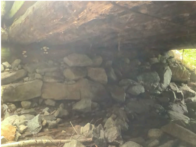
Left Bank Abutment when facing downstream
