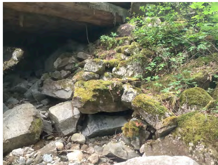
Left Bank Abutment when facing downstream
